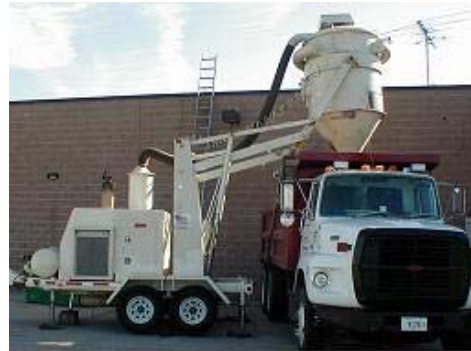
Mini-VecLoader Loading into a Dump Truck
