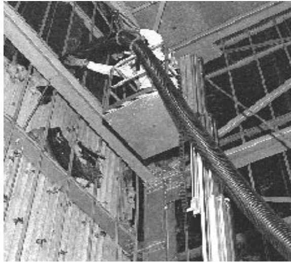
Figure 3. Worker removes insulation using the VecLoader HEPA vacuum system.
