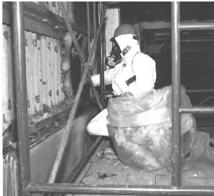
Figure 1. Worker manually removing insulation from walls.
